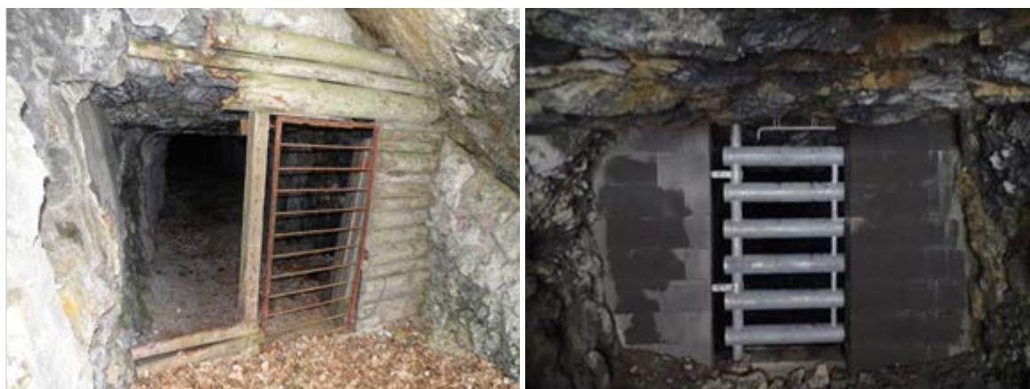
Fig.C6_1: Reconstruction of the entrance closure – locality Veľké prepadlé, SKUEV Homol'ské Karpaty
